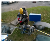
Fibre cable blowing in the new trench in Meyrin
