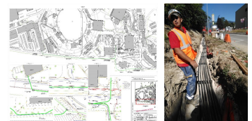
Optical fibre trench built in Meyrin
