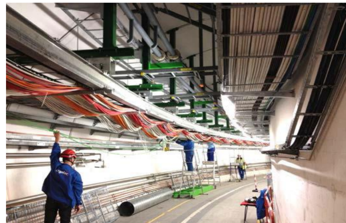
Typical cabling worksite
