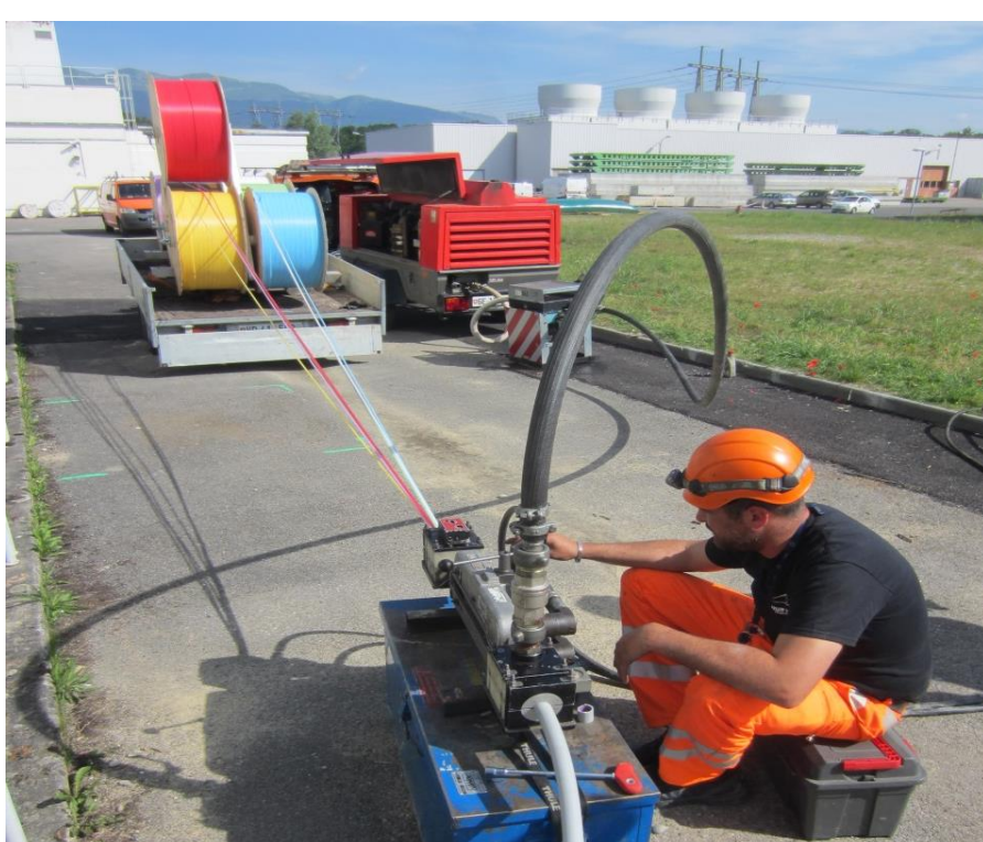
Optical cabling installation
